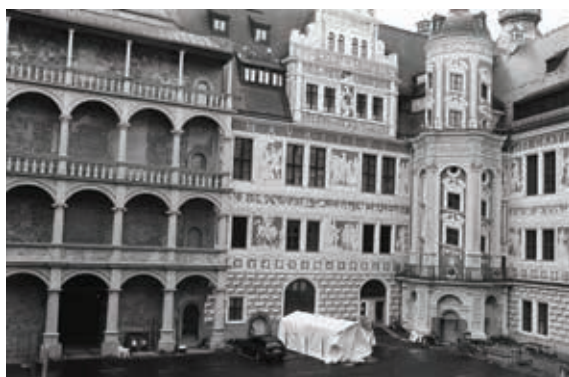
✓ Fig. 2. The main Residenzschloss courtyard under renovation, July 2016
