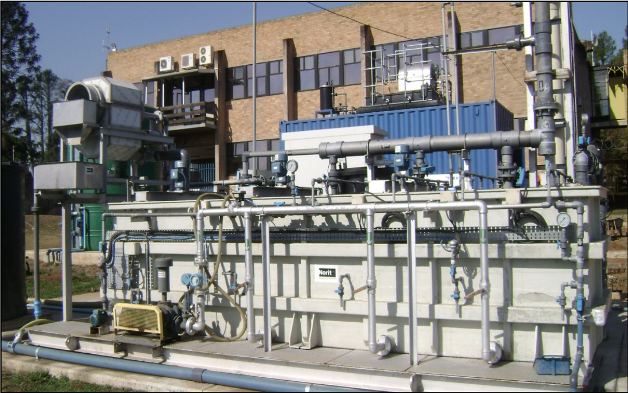
Figure 8 Norit MBR Pilot Plant showing Drum Screen (far left)
