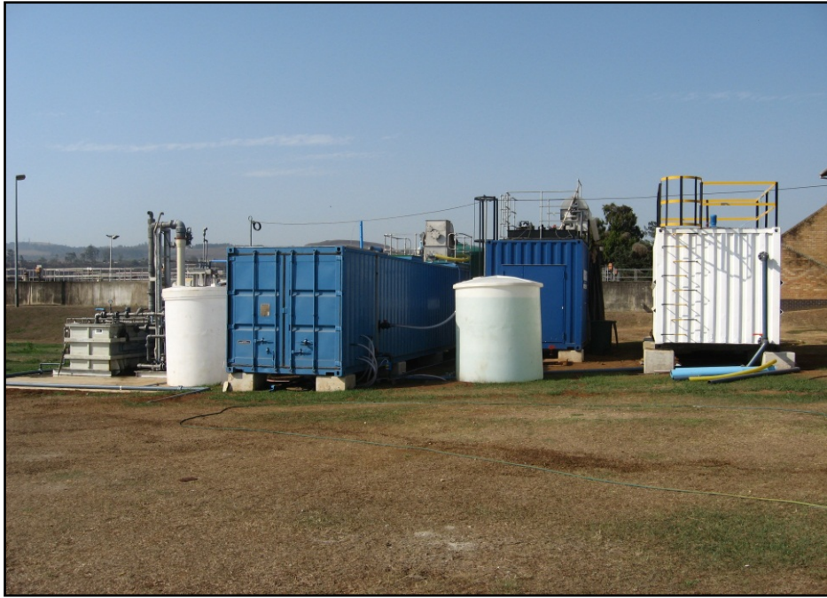
Figure 7: Onsite MBR Pilot Plant Set-up
