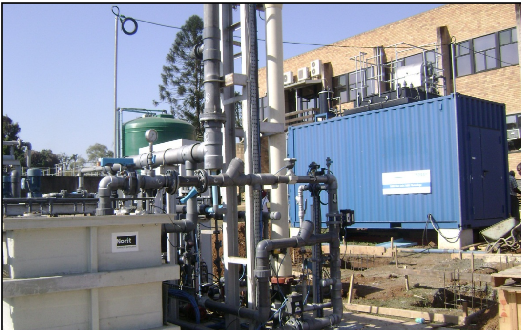
Figure 9: Norit MBR Pilot Plant showing External (Vertical) Membrane Module
