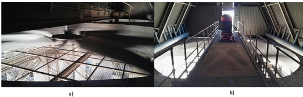
Figure 1.4: ACC unit in operation with (a) fan and (b) induction motor
