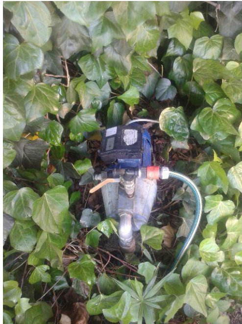
Figure A-3 Pump-pipe system: Environment C
