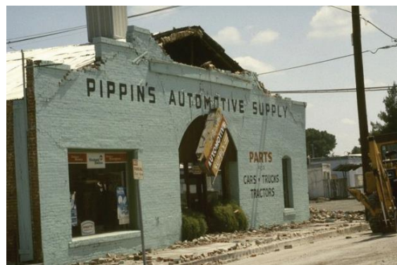
Figure 6: URM building with gable failure during Coalinga Earthquake of 1983 (Reitherman, 2009)
