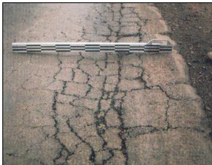
Figure 2. 4 - Cracking of the asphalt due to fatigue (TMH 9, 1992).
