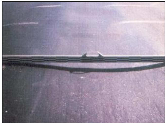
Figure 2. 2 - Severe condition of permanent deformation (TMH 9, 1992).
