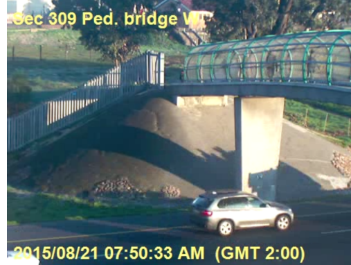
(f) Pedestrian bridge at camera 309 on the R300 with the camera facing West
