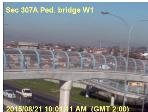
(d) Pedestrian bridge at camera 307A on the R300 with the camera facing West
