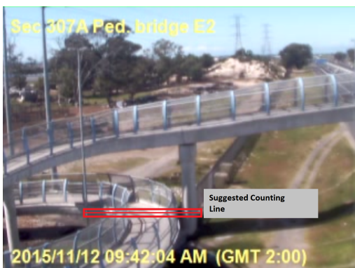
(c) Pedestrian bridge at camera 307A on the R300 with the camera facing East
