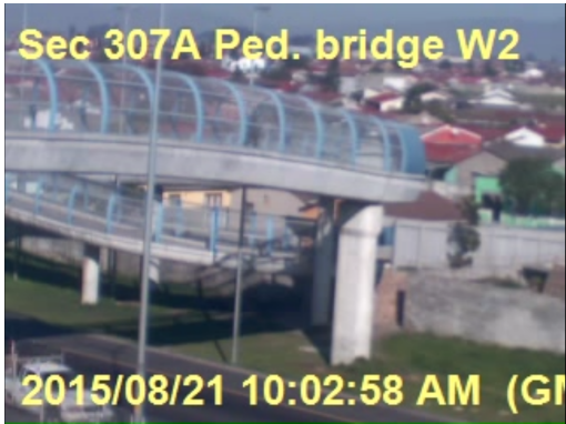
(e) Pedestrian bridge at camera 307A on the R300 with the camera facing West
