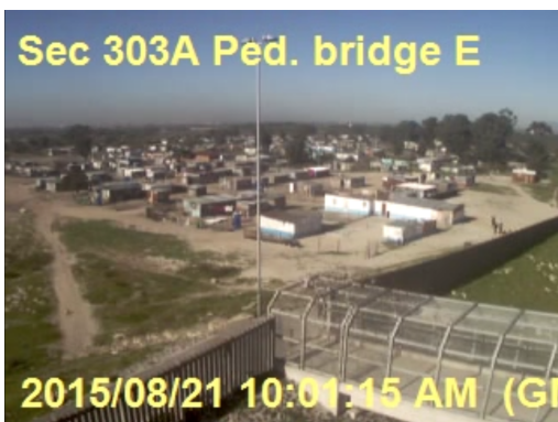
(a) Pedestrian bridge at camera 303A on the R300 with the camera facing East
