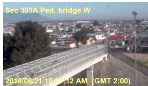
(b) Pedestrian bridge at camera 303A on the R300 with the camera facing West
