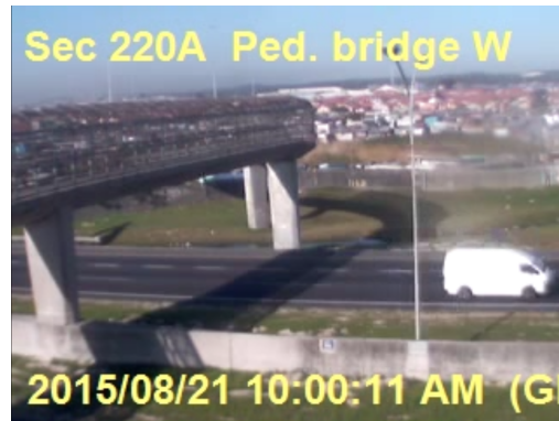
(h) Pedestrian bridge at camera 220A on the N2 with the camera facing West
