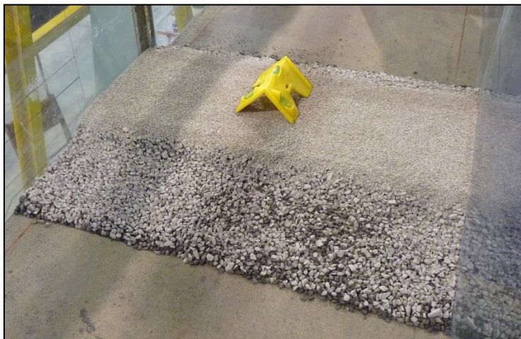
Figure C2: Levelling of screed layer
