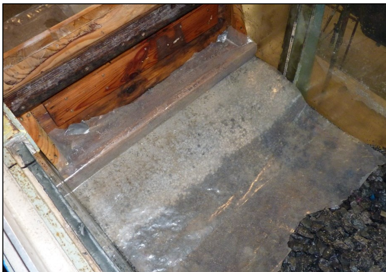
Figure C6: Plastic lining at back of structure
