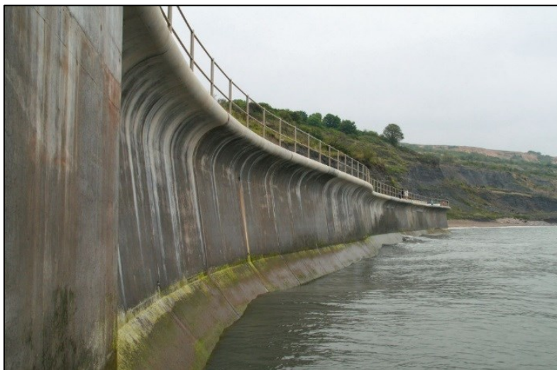
Figure 1: Vertical Seawall (Ian West, 2015)
