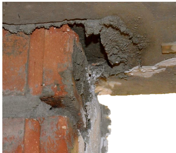
Figure A.10: SW-110-30-2 Top beam sliding failure.
