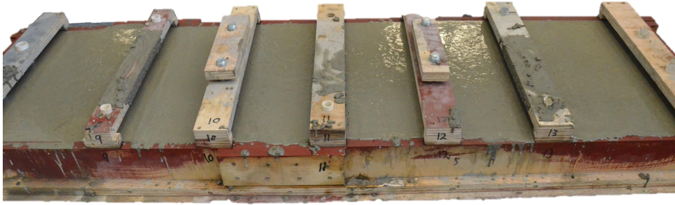
Figure 4.9: Freshly cast SCC used for top and bottom beams.
