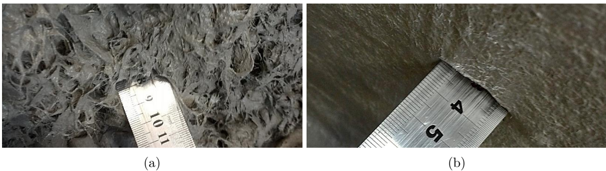
Figure 3.4: (a) 80 mm thick SHCC spray on thickness before trowelled flat; (b) 32 mm SHCC overlay, with good adhesion and no run down.
