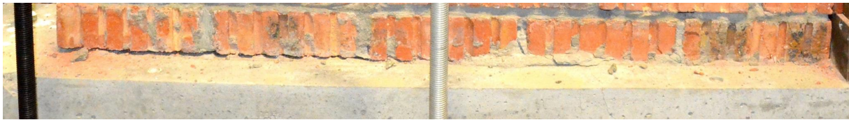
Figure A.9: SW-110-30-2 Flexural crack opening.
