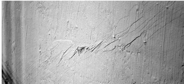
Figure 5.31: SW-220-15-3, Localized diagonal shear crack starting to form (before peak resistance was reached).
