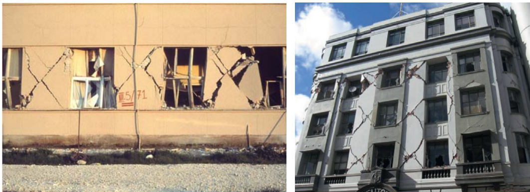
(a) Typical diagonal cracks in bottom storey. (b) Multi-storey building after earthquake.
