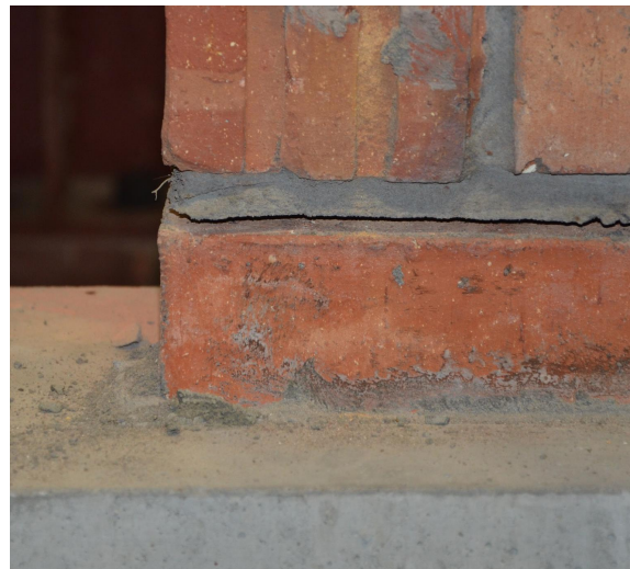
Figure D.2: Flexural crack opening.
