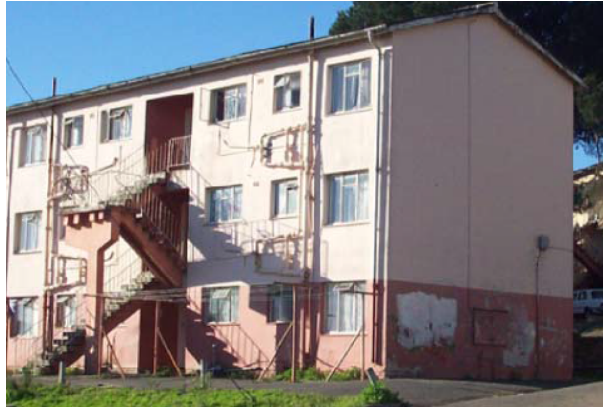
Figure 2.2: Typical URM building in the Cape Flats.
