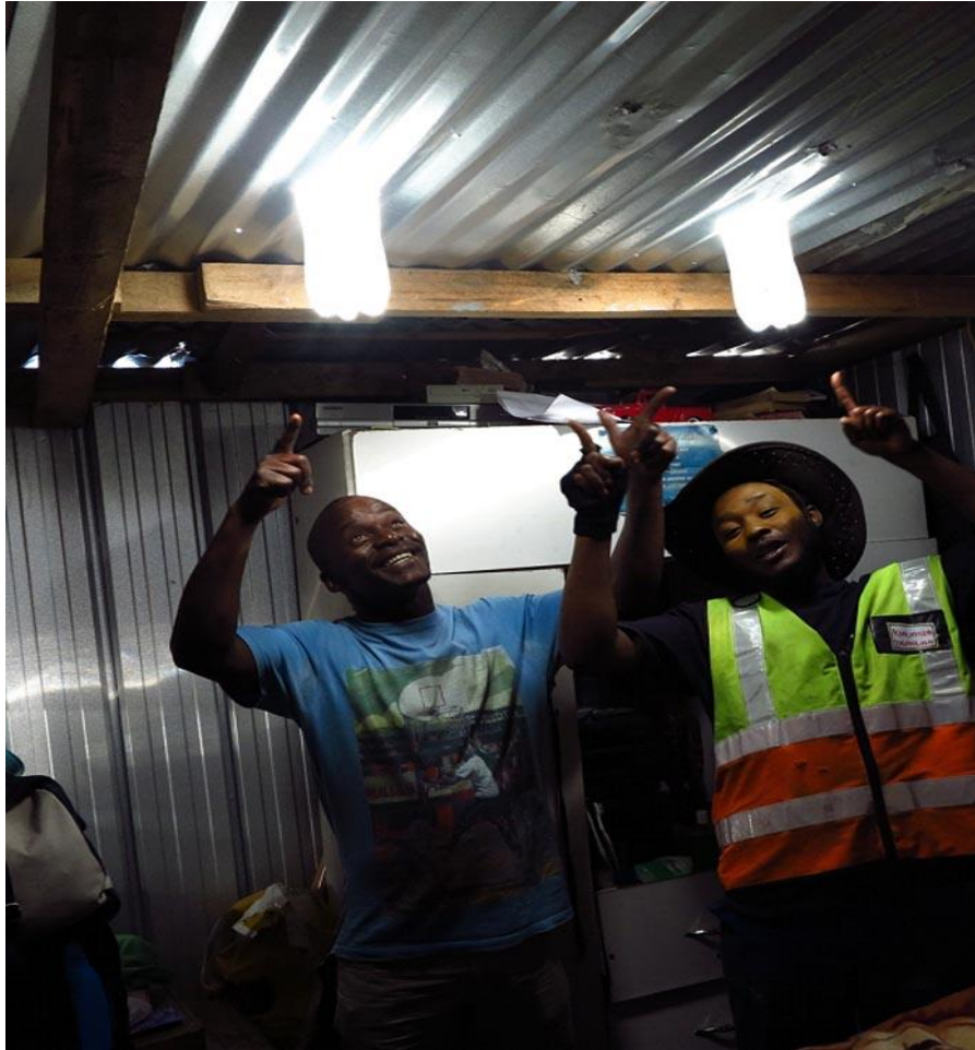
Photograph 4: Solar bottle bulbs installed in an informal household in Joe Slovo township in Cape Town Source: Mahala, 2012
