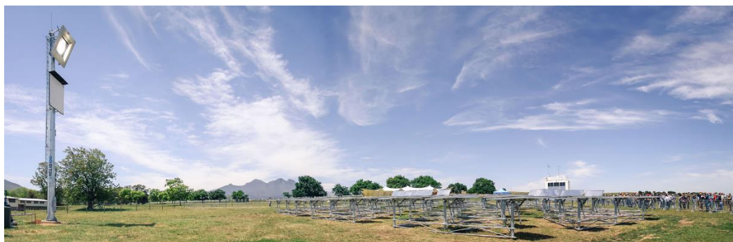
Figure 8.3: Helio100 central receiver pilot at Stellenbosch University (photo of SolarPACES 2015 technical tour courtesy of Helio100 project)
