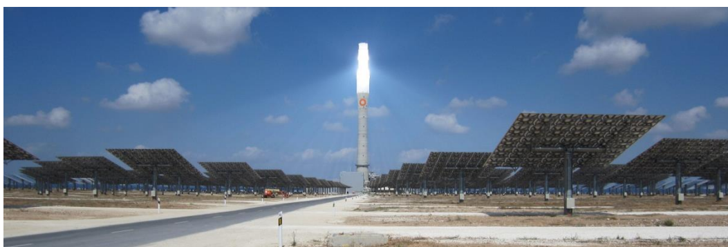
Figure 2.9: Gemasolar CSP plant, a 20 MW central receiver with 15 hours of storage (photo by author)
